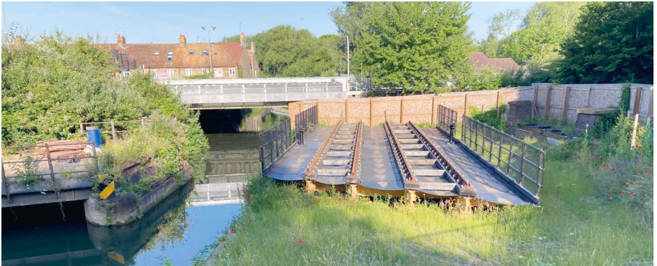
The Rewley Road Swing Bridge restored
